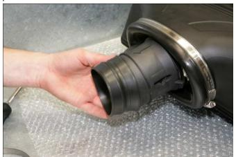
Secure with screw clamp. Note: for neatness ensure clamp head is in correct position
